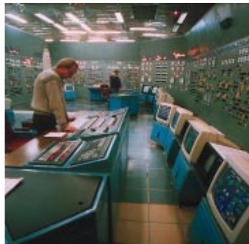
Two types of simulators were developed for training purposes at Soviet-designed nuclear power plants—analytical and full-scope simulators. U.S., Ukrainian and Russian organizations are working together to ensure each simulator replicates the configuration and behavior of each reactor.
