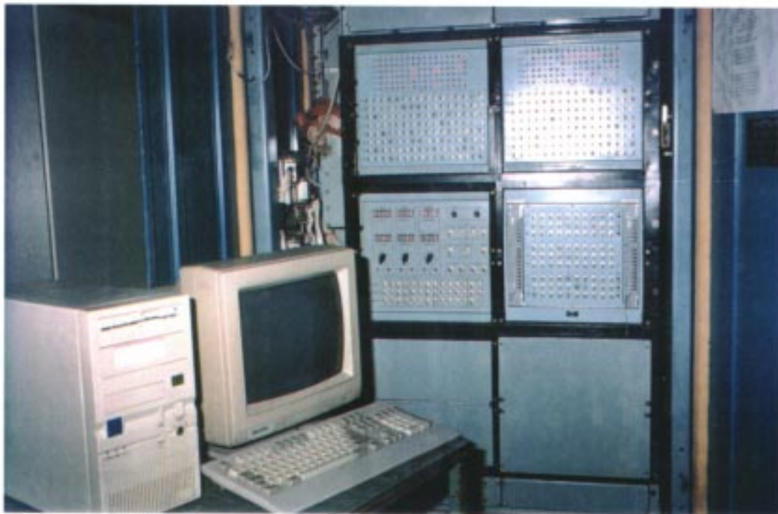
Adjustment means of CPT (Turbine regulation system)
