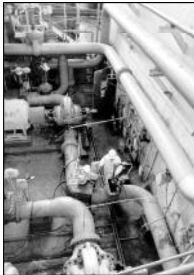
Reliability data on systems at Soviet-designed reactors will be collected in a central database and distributed first to six pilot plants and eventually to all plants with Soviet-designed reactors in nine countries to improve preventive maintenance. Left, 400-mm piping system in the turbine generator building at Smolensk NPP. Right, electric isolation valves in the ventilation system at Kola NPP.
