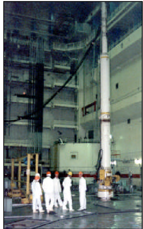
Spent fuel is removed from Chornobyl Unit 1.
